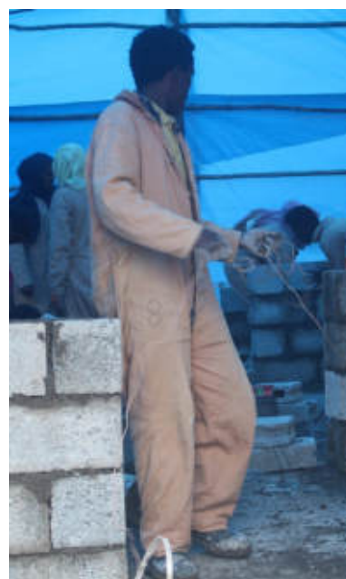
Figure 5. Short-term technical construction training
