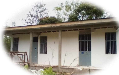
Butajira TVET college day care center under construction
